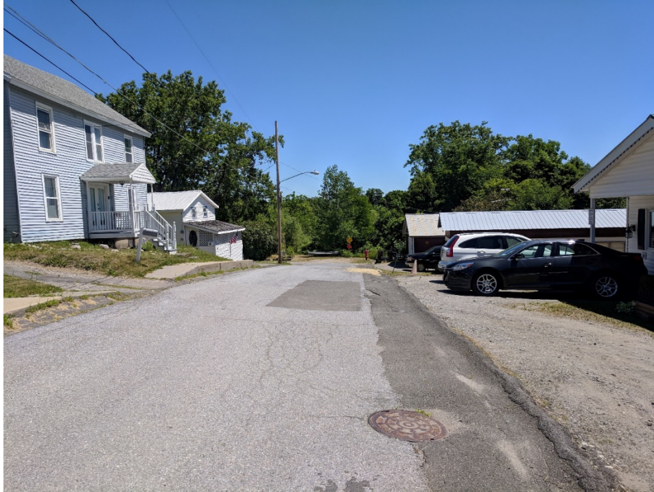
Figure 5: Water Main in Same Trench as Sanitary Sewer Not Meeting Design Standards
