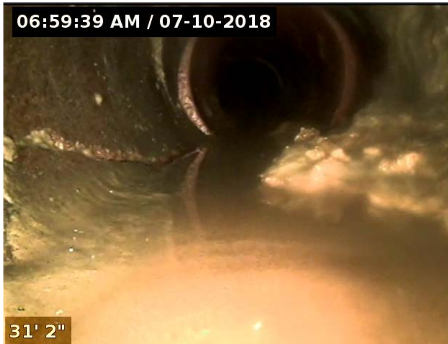
Figure 1: Broken Clay Sanitary Sewer Pipe 1
