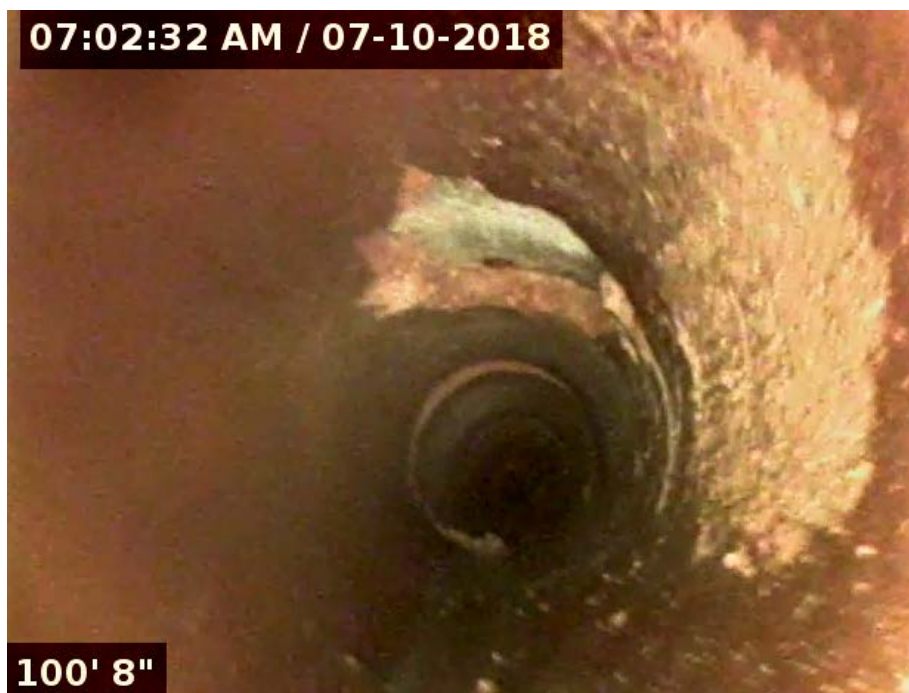
Figure 2: Broken Clay Sanitary Sewer Pipe 2
