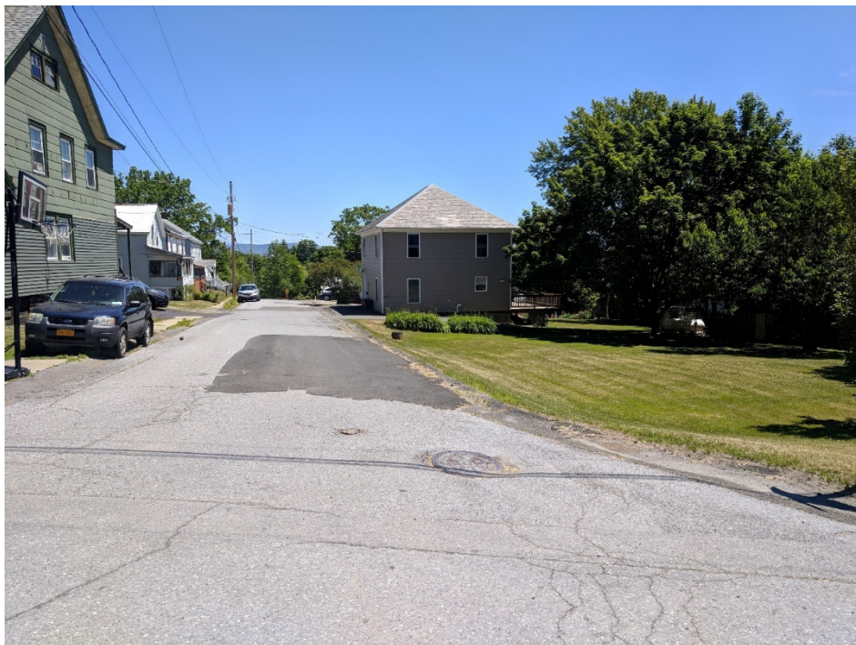
Figure 6: Water Main Valve Located in Close Proximity to Sanitary Sewer Manhole and Main
