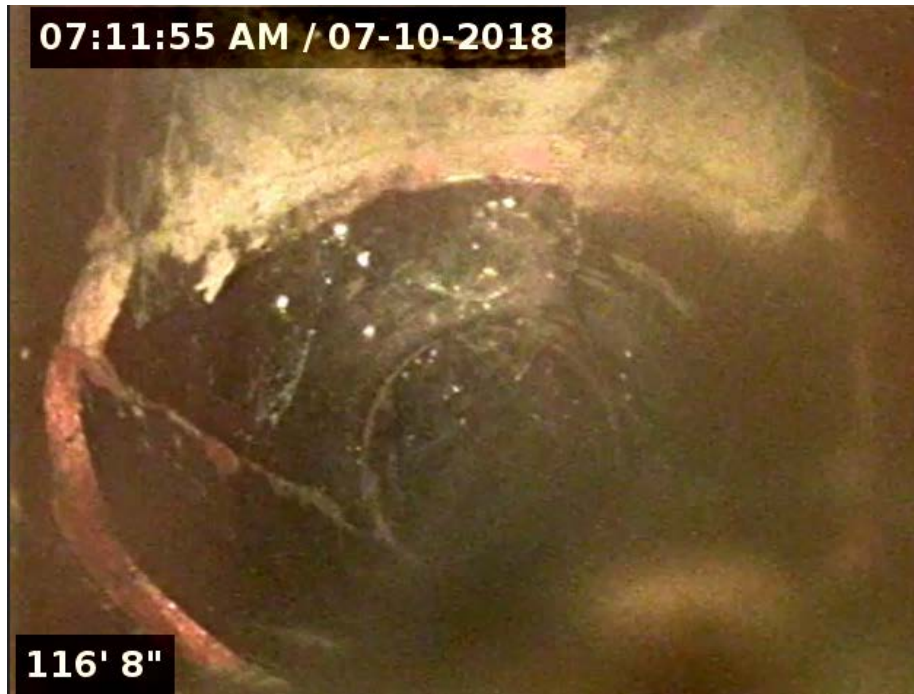
Figure 3: Failing Clay Sanitary Sewer Pipe
