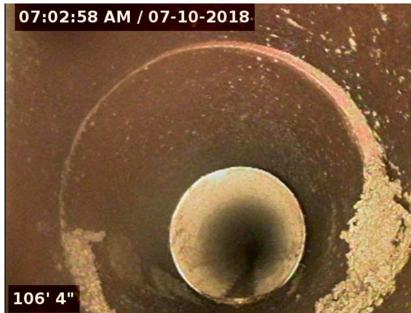
Figure 4: Joint Offset in Sanitary Sewer Pipe
